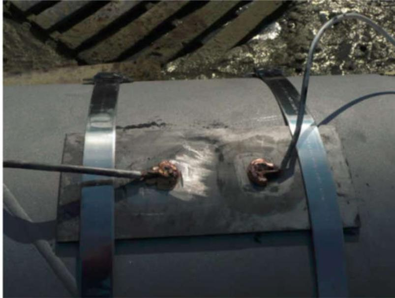
**Figure 6-8 Example of a Saddle Connection to a Pipeline**
