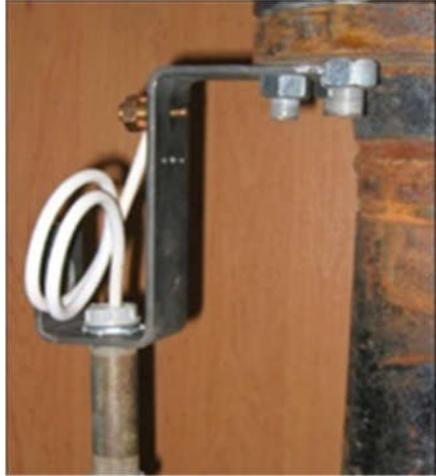
**Figure 6-2 Example of a Protective Bracket with Frost Loop, Servit Post™ and Frost Loop (a.k.a. pigtail)**
