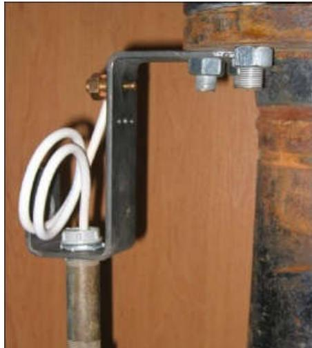
**Figure 5-1 Example of a Protective Bracket with Frost Loop and Servit Post™<sup>1</sup>**
