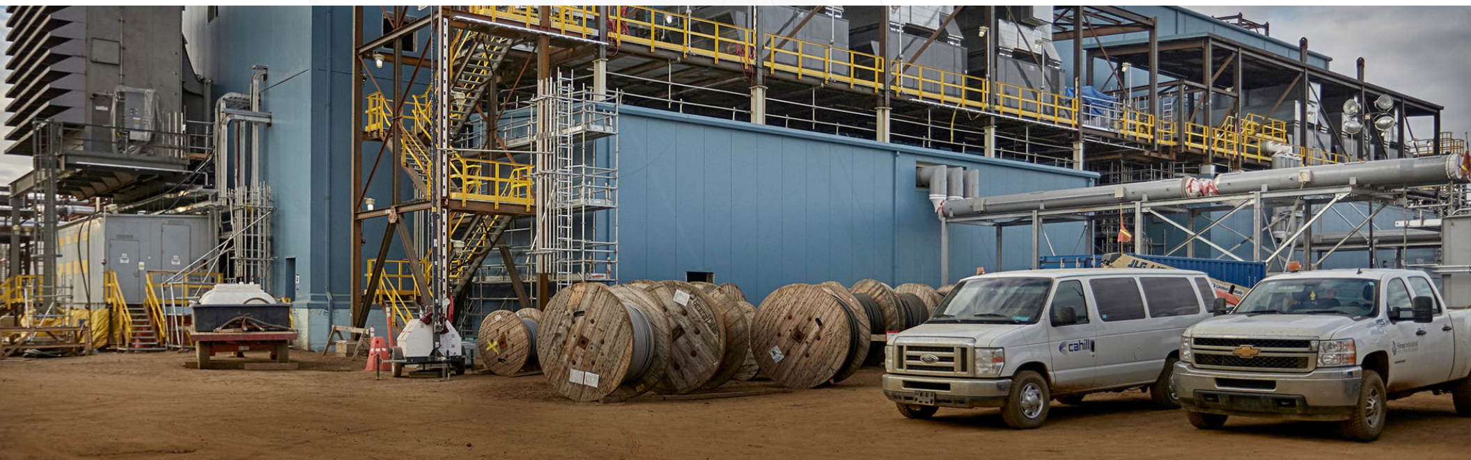
Cogeneration facility at Fort Hills. Photo courtesy Suncor.
