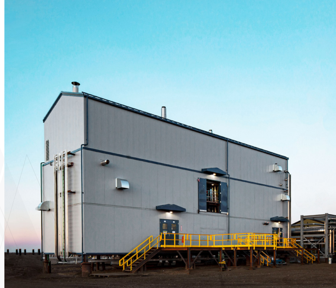
Carbon capture demo plant. Photo courtesy Svante.
