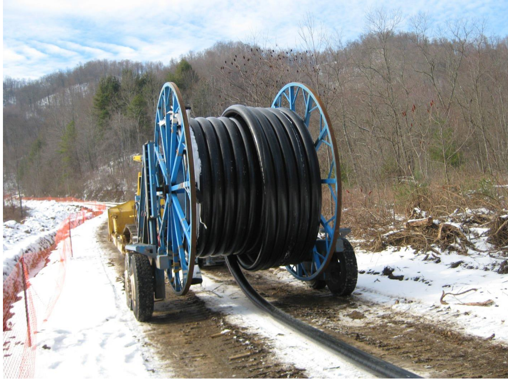
Figure 7-3 Spoolable Pipe Transport on Reel Trailer (Photograph courtesy of FlexSteel Pipeline Technologies Ltd.)
