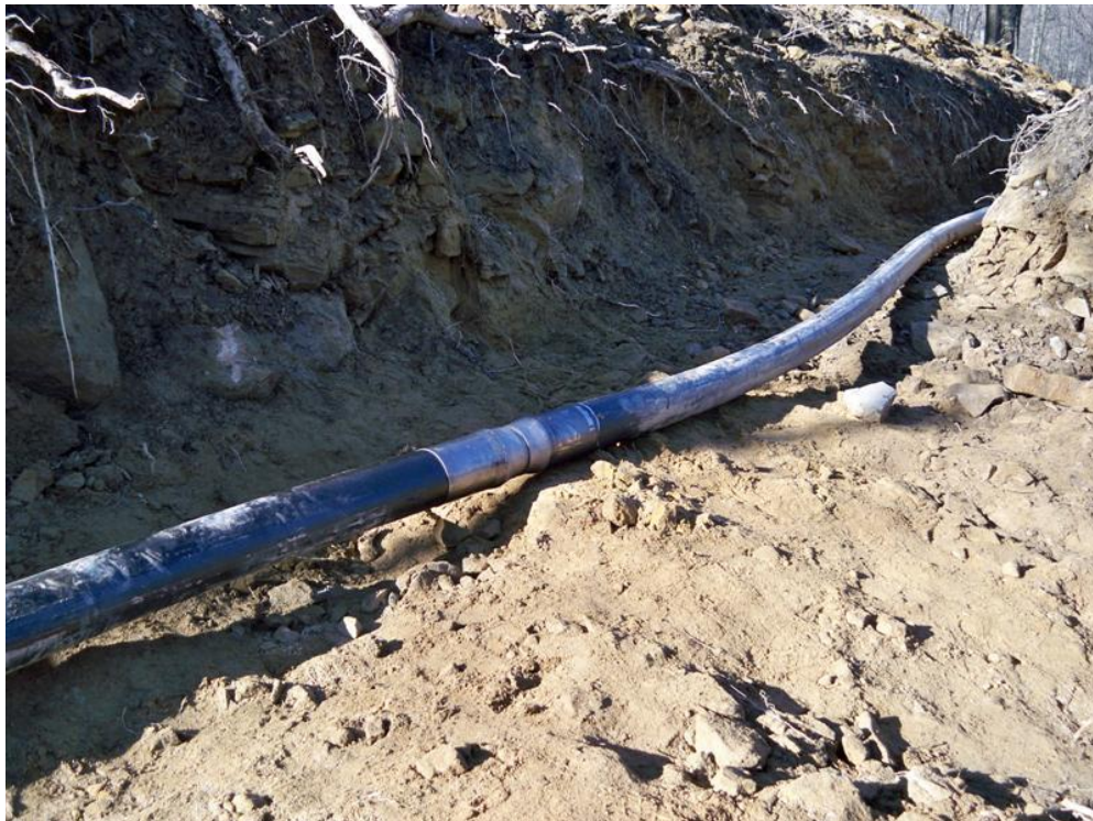
Figure 8-2 Metallic Coupler Joining Sections of Spoolable Pipe (Photograph courtesy of FlexSteel Pipeline Technologies Ltd.)
