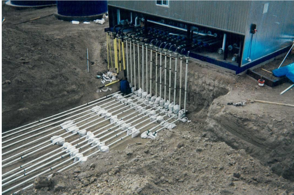
Figure 4-1 Pipeline Riser showing use of Sand Bagging for Support and Thrust Blocking. Composite Riser Extends above Grade to Flange Transition to Steel Piping (Photo used courtesy of Western Fiberglass Pipe Sales Ltd)
