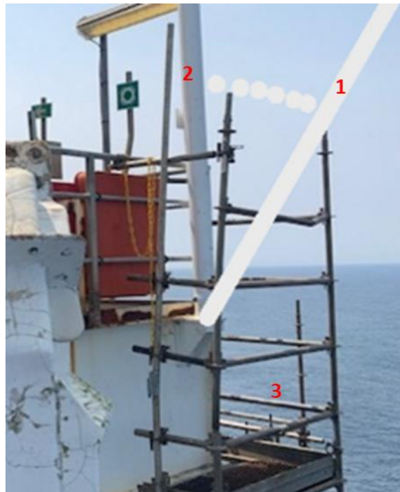
Fig. 1. Position of Light Pole and Scaffolding
